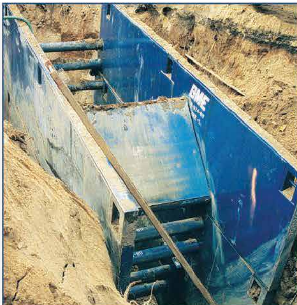
Special shield using a custom bedding slide.
