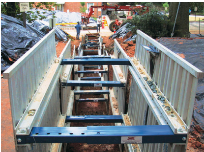
Hydraulic Aluminum Shield with End Loadable Struts R
