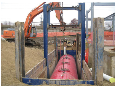
Slide Rail with Pit Configuration
