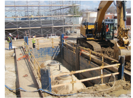
Clear Span Slide Rail with Tiebacks
