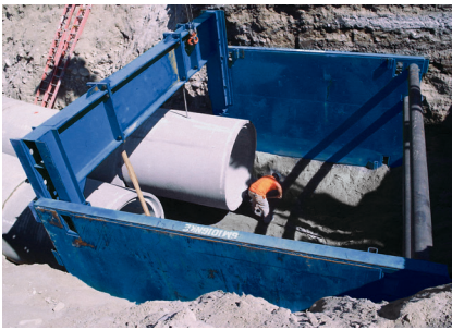
Height Adapter with Steel Trench Shield
